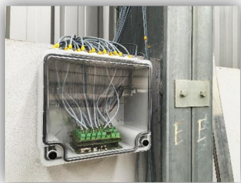
Figure 4 – Installation of data acquisition system.
