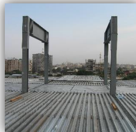
Figure 3 – Composite slab.
