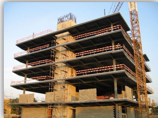
Figure 1 – New Rectory building of UCAN.
