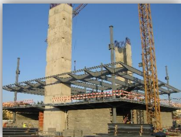
Figure 2 – Construction of 2 nd floor.
