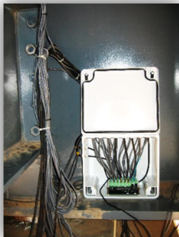
Figure 5 – Installation of data acquisition system.
