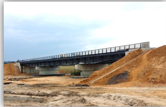
Figure 1 – Bridge over Uhamba river.
