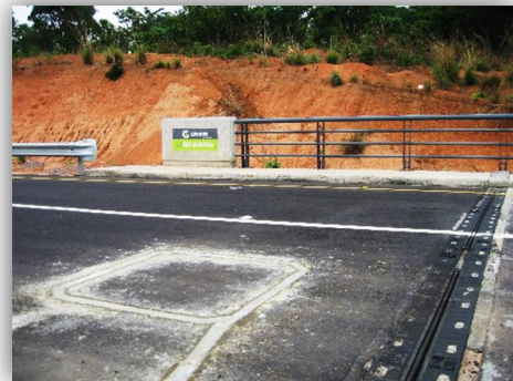
Figure 7 – Installation of inductive loop on the pavement for traffic detection.
