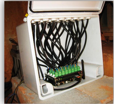
Figure 7 – Installation of the data acquisition system at the North abutment.
