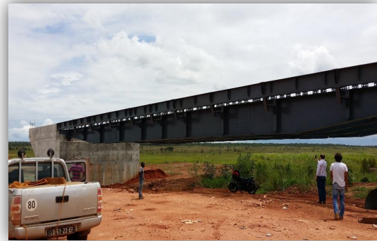
Figure 1 – Bridge over Kusso river.
