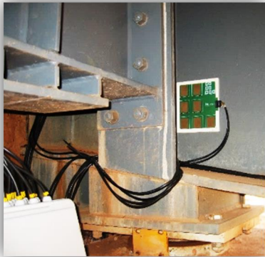
Figure 5 – Installation of the corrosion sensor at the North abutment.
