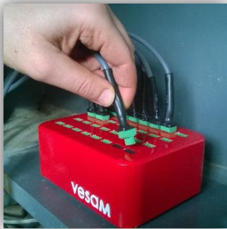
Figure 4 – Installation of data acquisition system.
