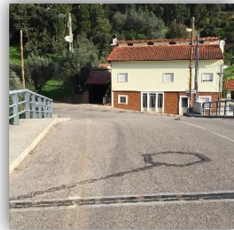
Figure 6 – Installation of inductive loop on the pavement for traffic detection.
